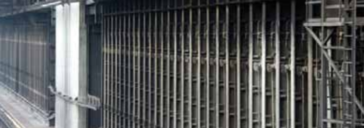
Coke oven battery
