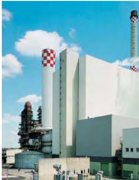
Industrial power plant
