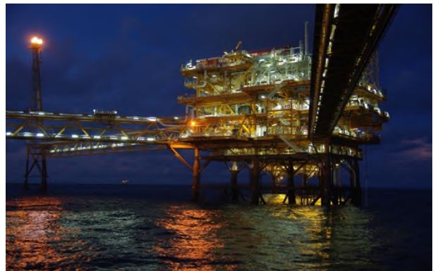
Fully automatic remote monitoring of oil platform movements and sea level under extreme offshore environment conditions.
