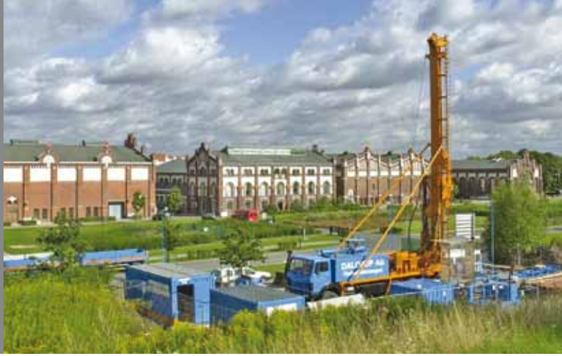
Drilling site in Waltrop, Germany
